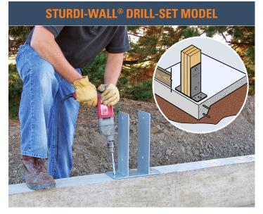
For applications in which the concrete foundation has already been poured and cured, use the Sturdi-Wall® drill-set model. It reduces costly placement errors when a concrete subcontractor is used. Installation is quick and easy, requiring only a hammer drill with masonry bit and concrete fasteners.
